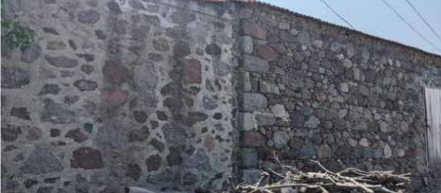
ESKİ VE YENİ DUVAR OLD AND NEW WALL
